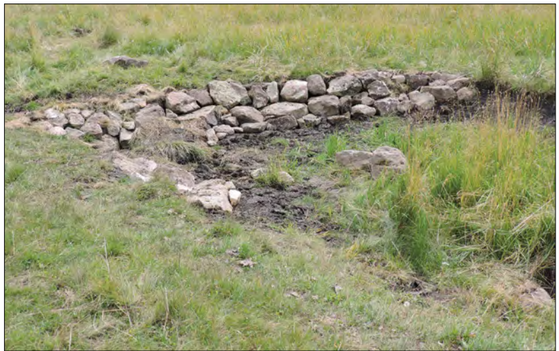
Figure 52. Site 11, August 25, 2015. Rock layback after construction. (©W.D. Zeedyk)
