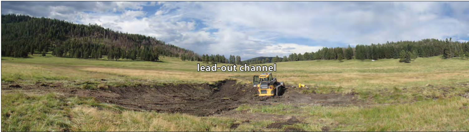
Figure 29. Sod has been added to cap the plug. Skid loader is constructing lead-out channel. (©S. Vrooman)
