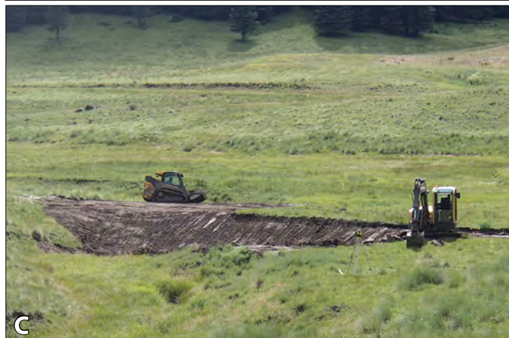
Figure 22. Site 52, August 3, 2016. A: Stockpiled sod. B: Excavator borrowing soil from pond. Skid loader is building and compacting the plug. Outlet in the foreground. C: Adding stockpiled sod to the surface of the plug. (©S. Vrooman)
