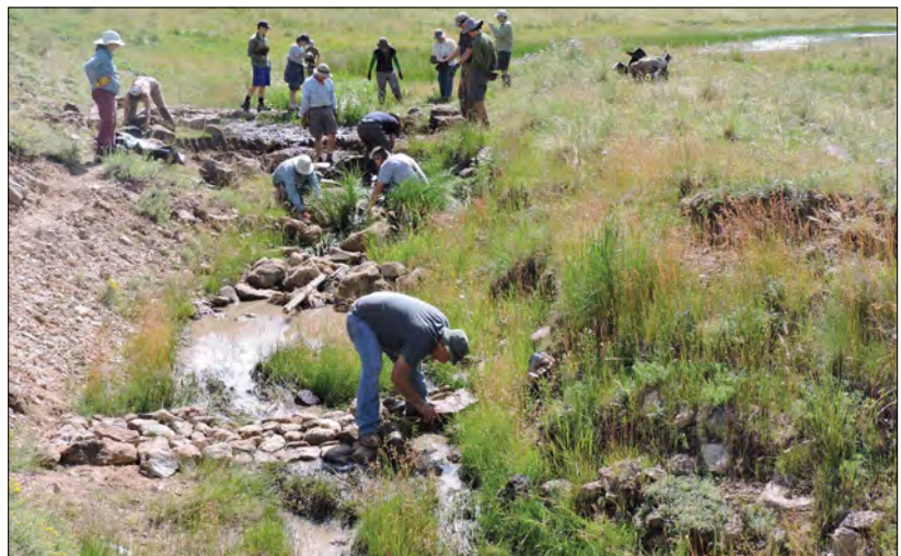
Figure 56. Site 50 and 51, July 18, 2015. Volunteers build grade control rock structures at stock pond outlet. (©W.D. Zeedyk)
