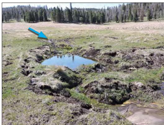
Figure 50. Site 38, left, sod Zuni bowl after construction, May 13, 2016 and right, one year later, May 11, 2017. (©W.D. Zeedyk)
