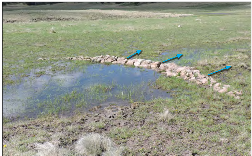
Figure 47. Complex Site 28, May 11, 2017. Media luna spreading water downvalley from plug and pond. (©W. D. Zeedyk)
