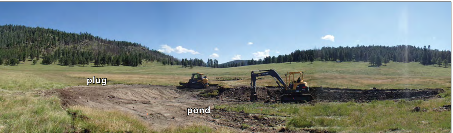
Figure 28. Constructing and compacting the plug. (©S. Vrooman)
