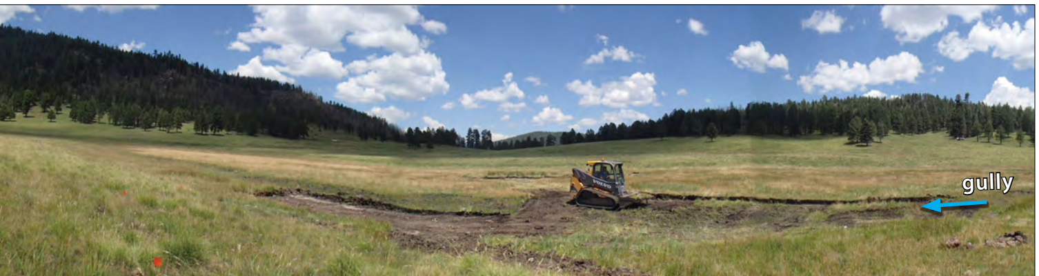
Figure 27. Excavator is removing sod from the surface of the area to be ponded and stockpiling it for surfacing the plug. (©S. Vrooman)
