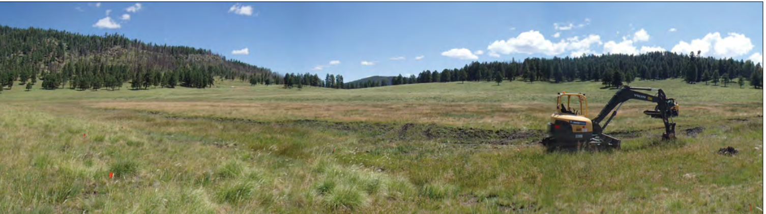
Figure 26. Beginning construction of the pond by borrowing fill for the plug. (©S. Vrooman)
