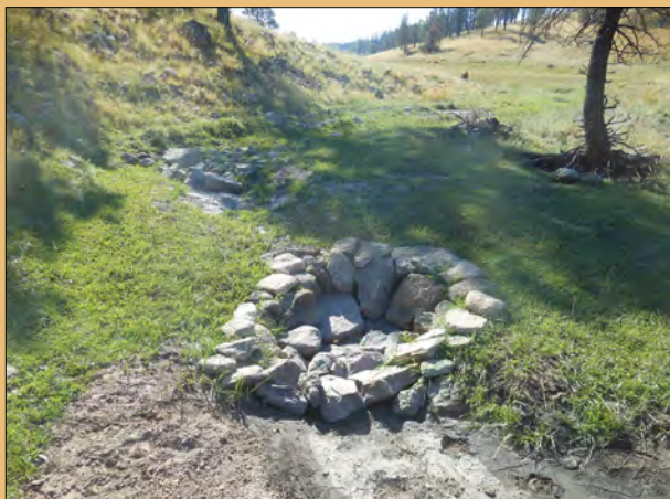
Figure 17. Left, rock headcut control structures, September 21, 2012. Right, same site now occupied by wet meadow vegetation October 2, 2017. (©S. Vrooman)
