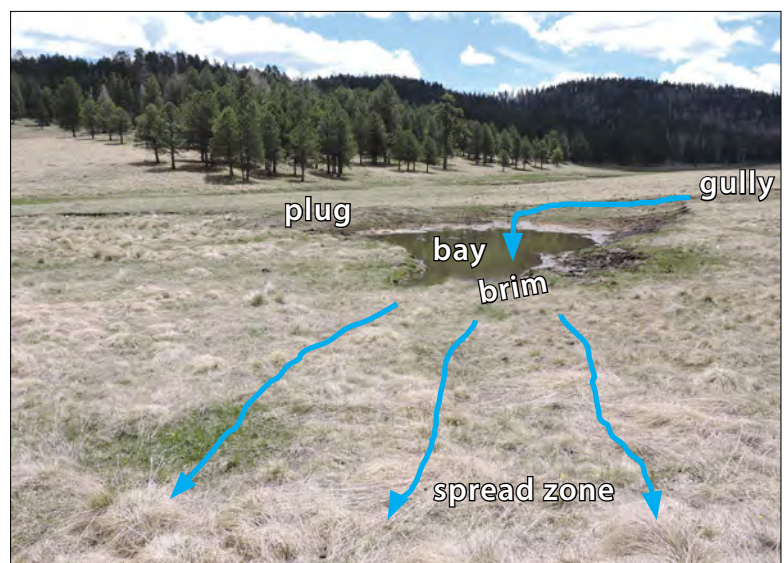
Figure 39. Site 18, May 11, 2016. Plug and spread treatment. (©W.D. Zeedyk)
