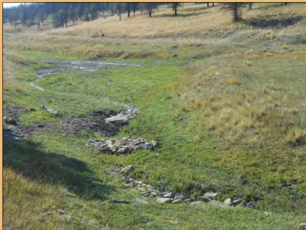
Figure 16. Left, small rock grade control structures, September 22, 2012. Right, same site now occupied by wet meadow vegetation, October 2, 2017. (©S. Vrooman)
