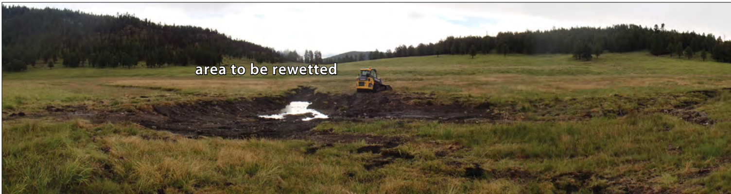
Figure 30. Pond beginning to fill as construction continues. Area to be rewetted is beyond the end of the lead-out channel. (©S. Vrooman)
