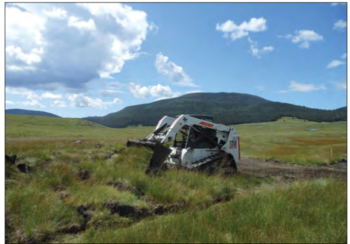
Figure 36. Tres Arroyos, August 2012. Left, skid loader adds fill dirt excavated from the pond to the surface of the plug. Right, sod tiles stockpiled prior to constructing the plug are placed on the completed plug. (©S. Vrooman)
