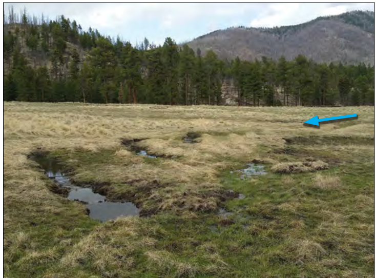
Figure 44. Site 31, April 20, 2017. Upper swale, left, diverts flow around a headcut and directs it to two spreader swales, valley left. (©S. Vrooman)
