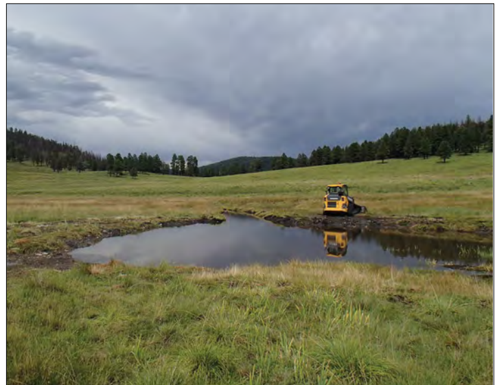
Figure 4. Site 21, August 7, 2016. A plug and pond on a perennial channel fills soon after construction. (©S. Vrooman)
