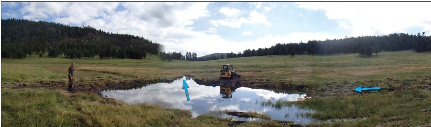
Figure 31. Construction completed and water from lead-out channel is spilling onto reconnected wetland surface. (©S. Vrooman)
