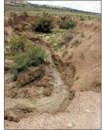
Gully on San Pablo Creek.
