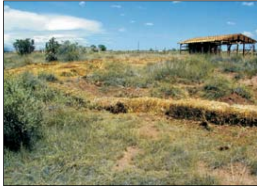
Strawbale headcut control on contour, Galisteo watershed, 2001.
